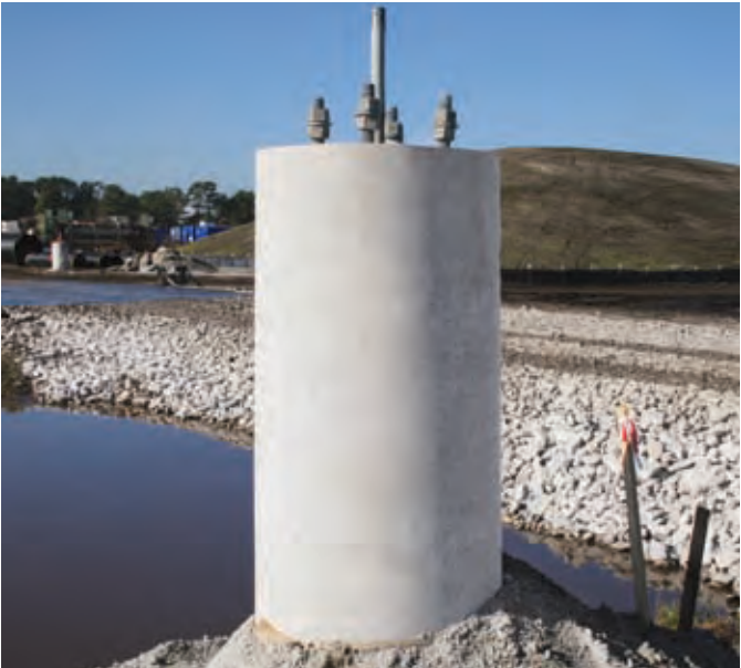
Sonotube Finish Free form column
